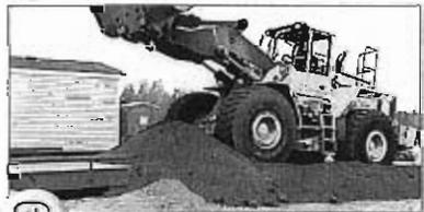
3 Backfill to bulkheads and finish ramps.
